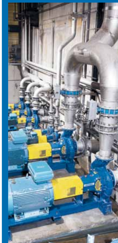
◀ Single-stage centrifugal process pumps (installed on PM1 at Myllykoski Continental GmbH in Plattling, Germany).
