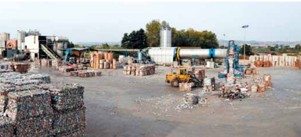
▲ The FibreFlow® Drum processing line at Alier. About 30-40 different grades of waste-paper are processed into a variety of paper products at the mill.
