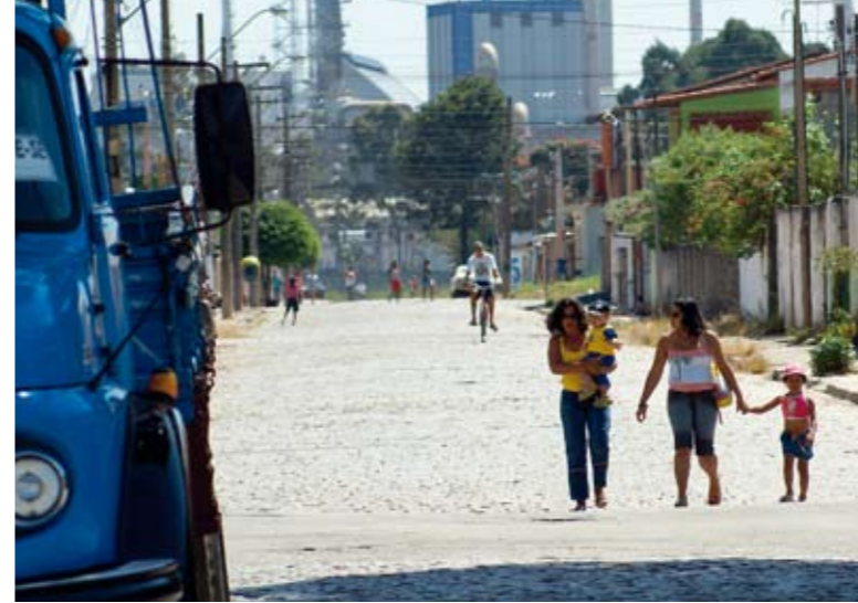
Good neighbors. Residents of Suzano walk the streets in front of their homes. In the background is one of the recovery boilers that now benefits from Andritz technology to reduce odor. ▲
