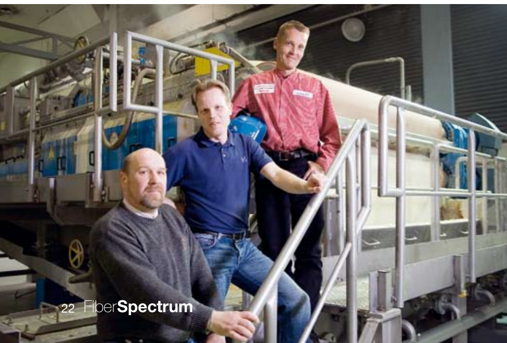
◀ Shown from bottom to top on the Andritz twin wire press in the new peroxide bleach plant are Vesa Holm, Supervisor, Harri Taipale, Production Engineer, and Jorma Latva-Kokko, Production Manager, at the Summa mill. In total, there are five such presses in the bleach plant, which is designed to produce 560 adm/d of 80+ ISO brightness on TMP grades.
